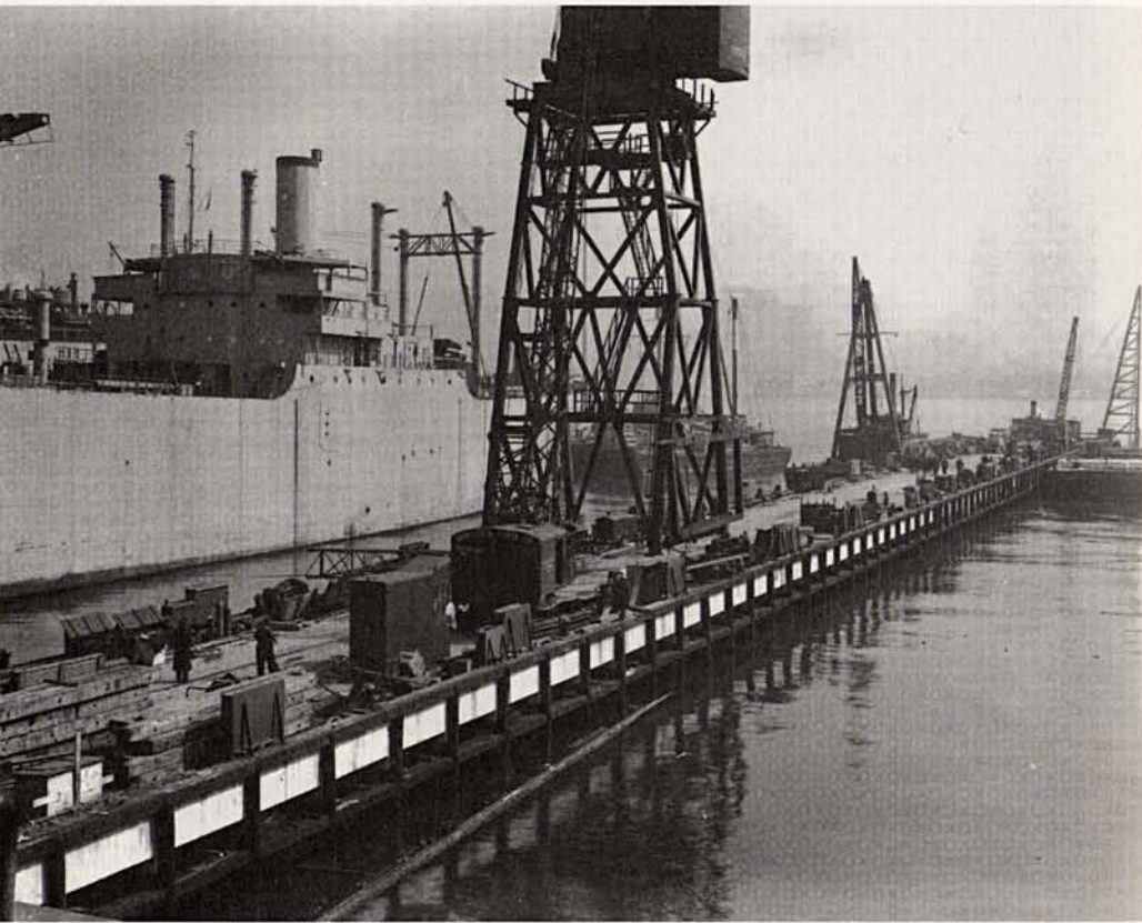
Gantry crane on Hoboken pier, 1944.
