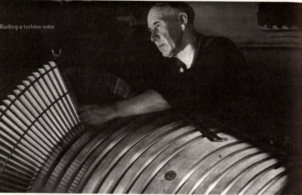
Blading a turbine rotor in the Bethlehem Steel Shipyard Machine Shop, photo circa 1940. Included in a company brochure found on the property in 1990.
