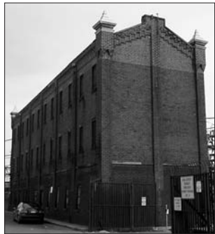
Record Building at the foot of Washington St.
